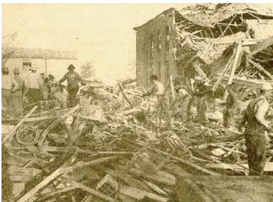
Picture of the schoolhouse after the explosion
